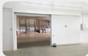
Plant of heating equipment «FerroliBel», Minsk region Retractable fireproof gates «FireDoors» Ei60
